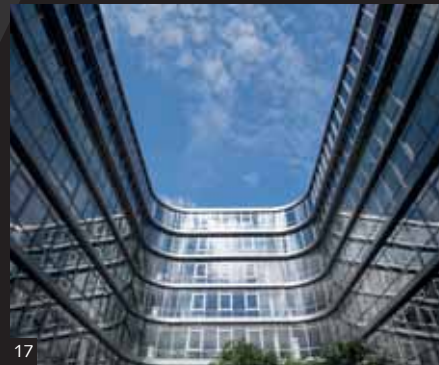
Siemens Headquarter Munich/Germany
