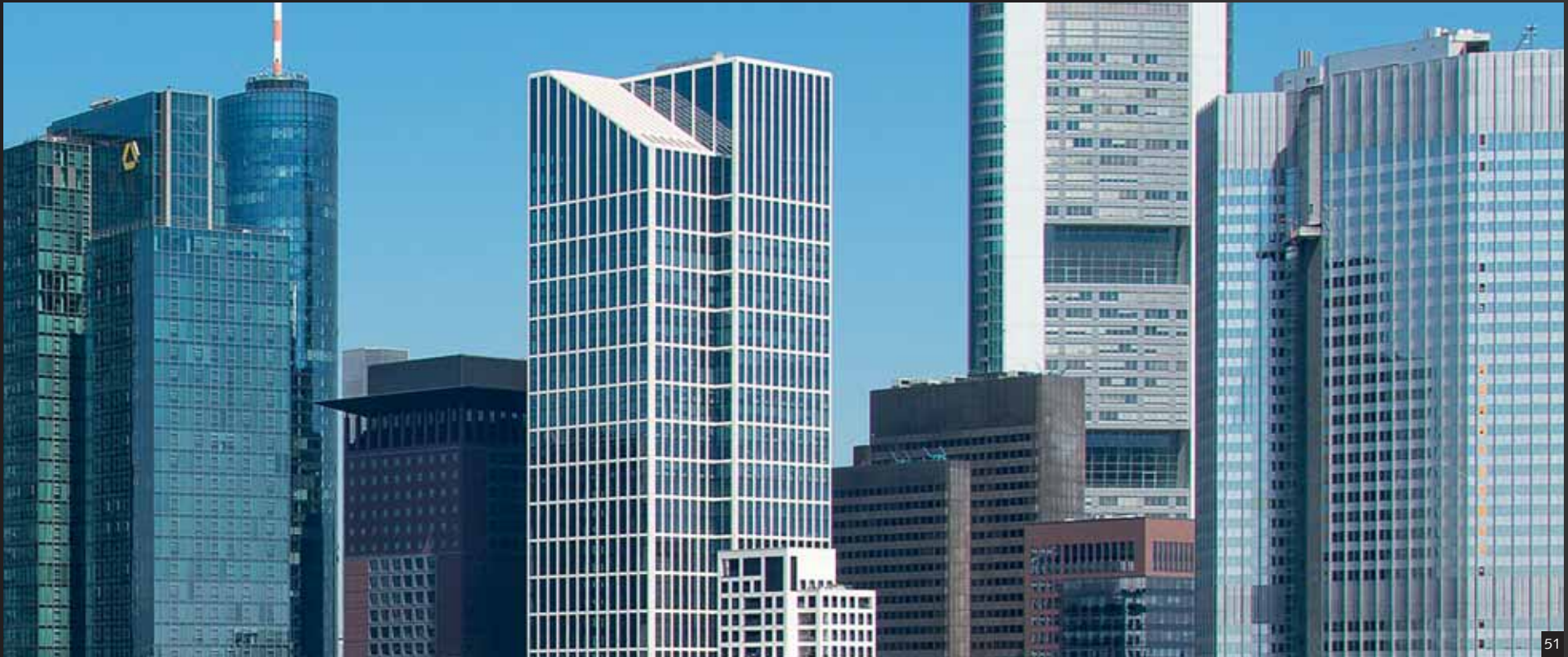
Taunusturm, Frankfurt Main/Germany
