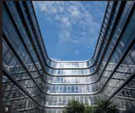
Siemens Headquarter Munich/Germany
